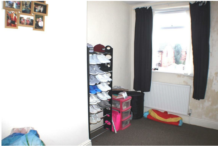
Rear aspect window and radiator.
